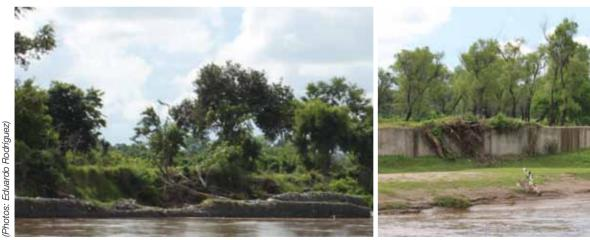
The levee built in 2006 is seen destroyed (left), or submerged in the rising waters of the Paz River (right).
