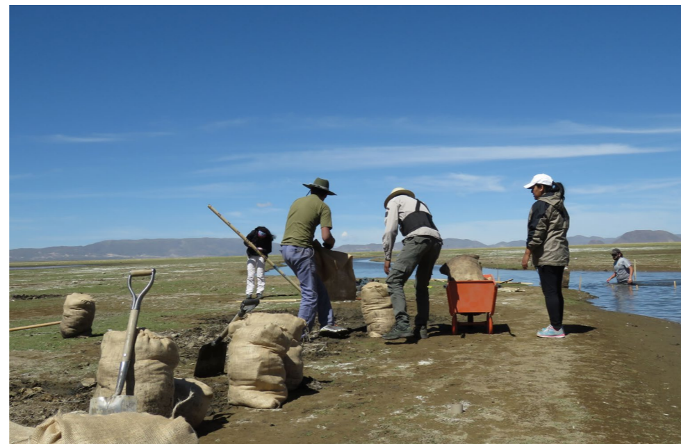
Construction work Rio Chico
