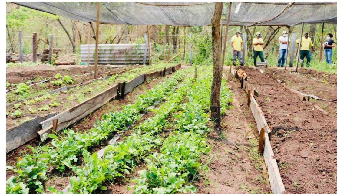
Construction of nursery space and community garden Kadiwéu
